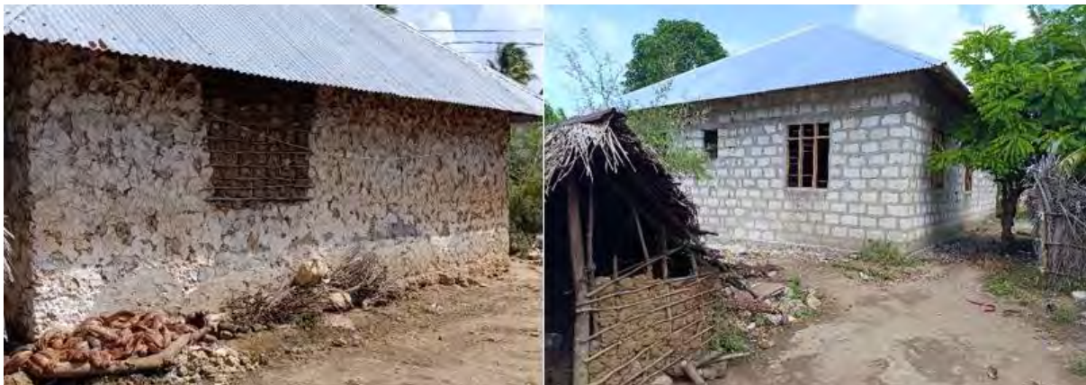
Plate 1 Building materials from mud, limestone to cement block-quality check
